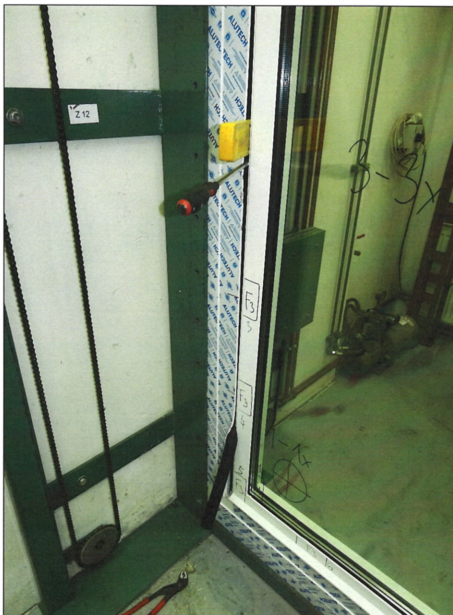
Pic. 11 – test sample No. 15/2023-1 after manual test No. 4 (view from the side of the attack – outside)
