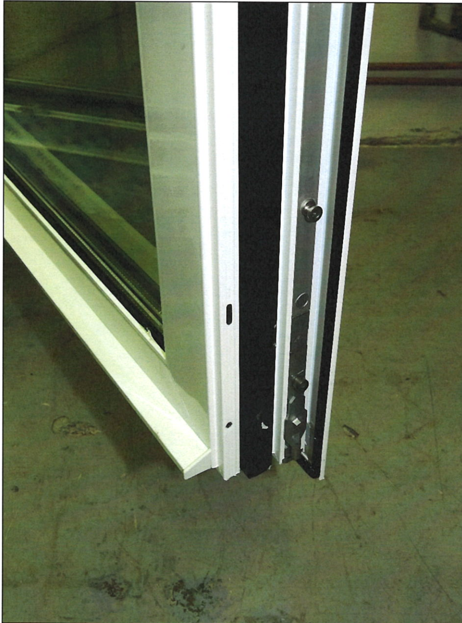
Pic. 5 – detail of locking pins
