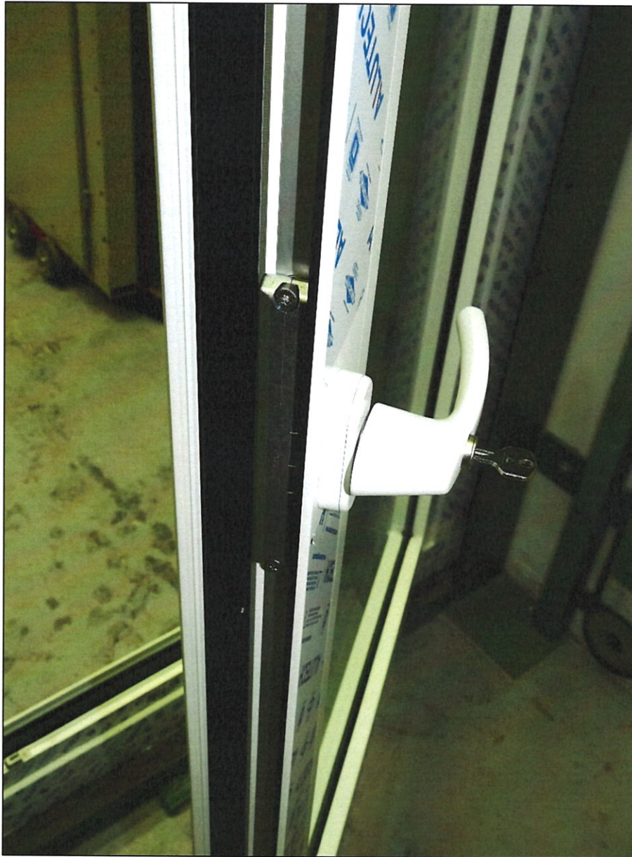
Pic. 4 – detail of key operated lockable window handle Roto Line – lockable window handle 200 Nm
