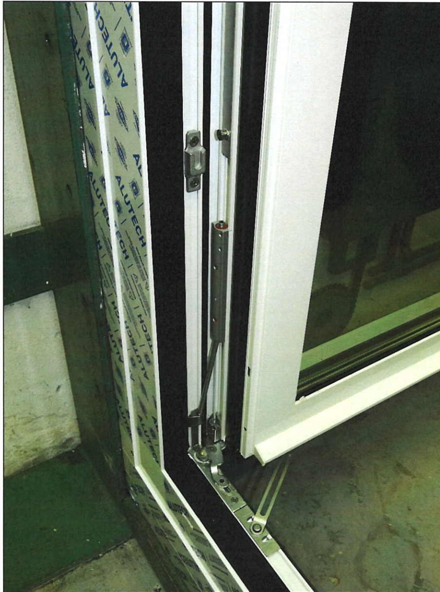
Pic. 2 – detail of lower hinge and locking pins
