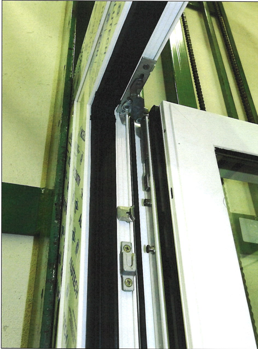
Pic. 3 – detail of upper hinge and locking pins
