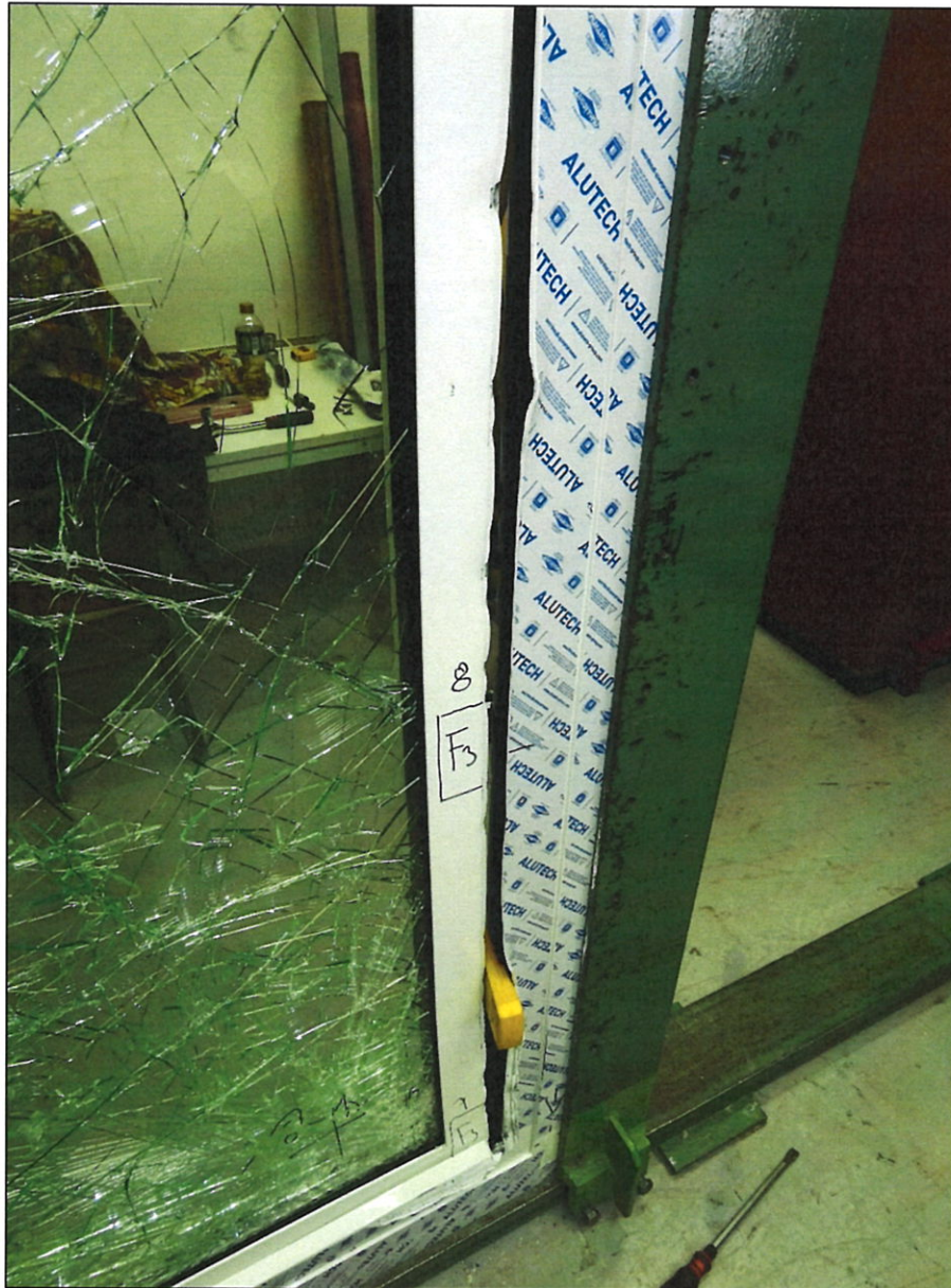
Pic. 10 – test sample No. 12/2023-1 after manual test No. 3 (view from the side of the attack – outside)
