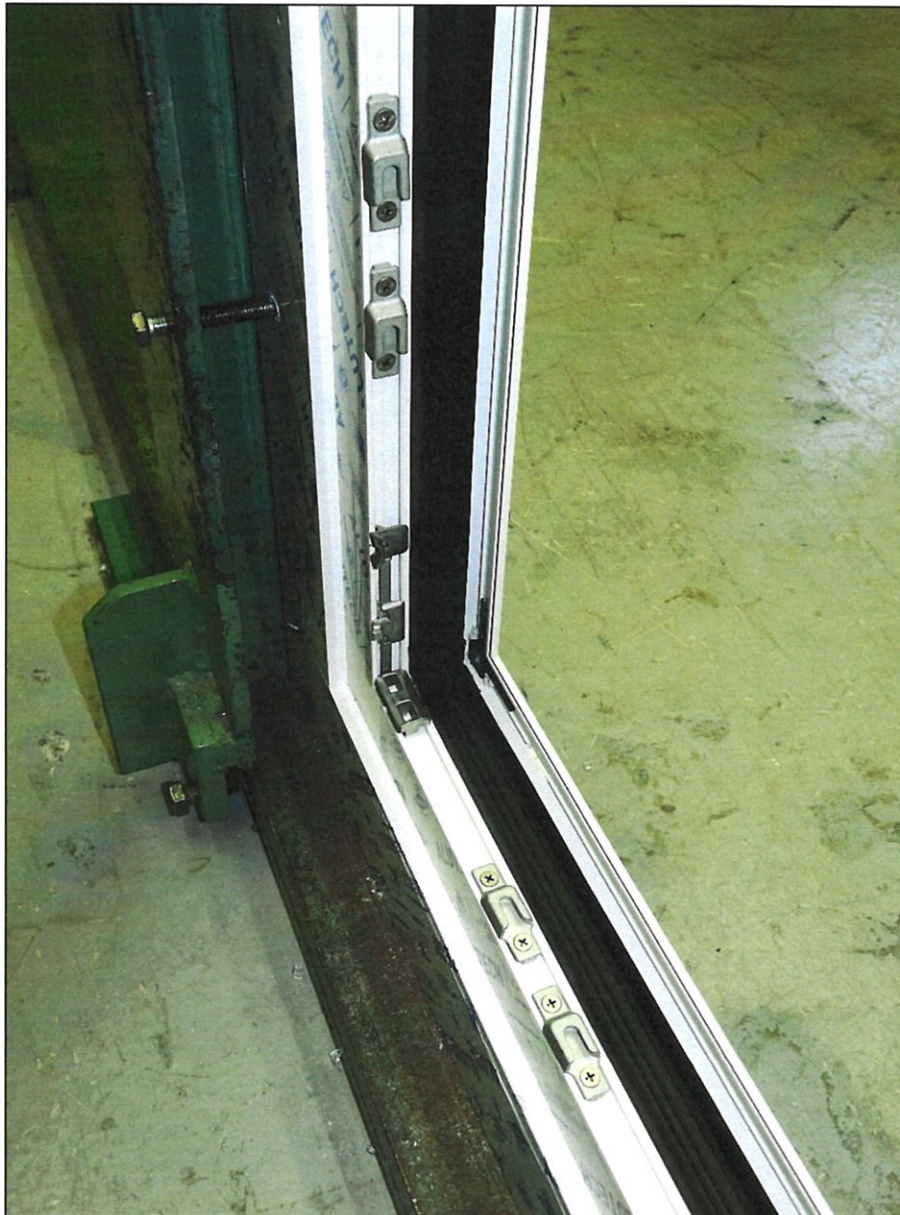
Pic. 6 – detail of fitting holes for locking pins
