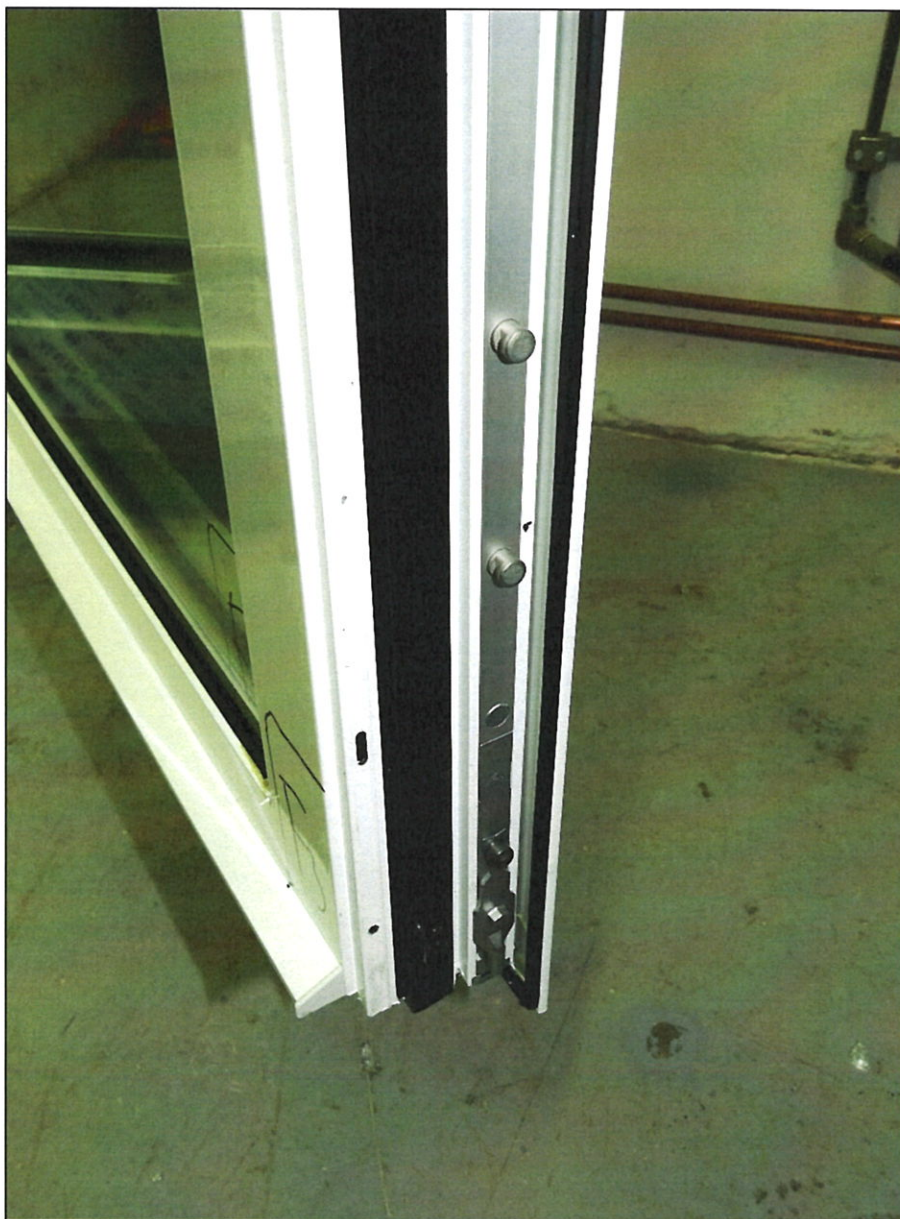
Pic. 5 – detail of locking pins
